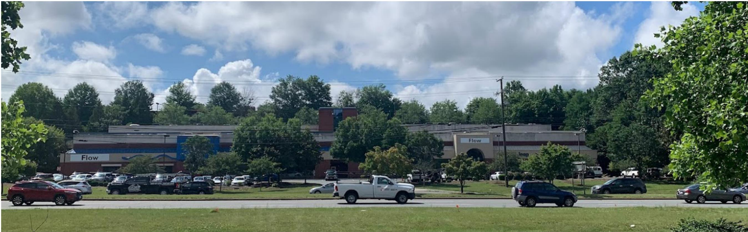
04 VIEW-FROM EAST OVER STREET - WHOLE BUILDING
